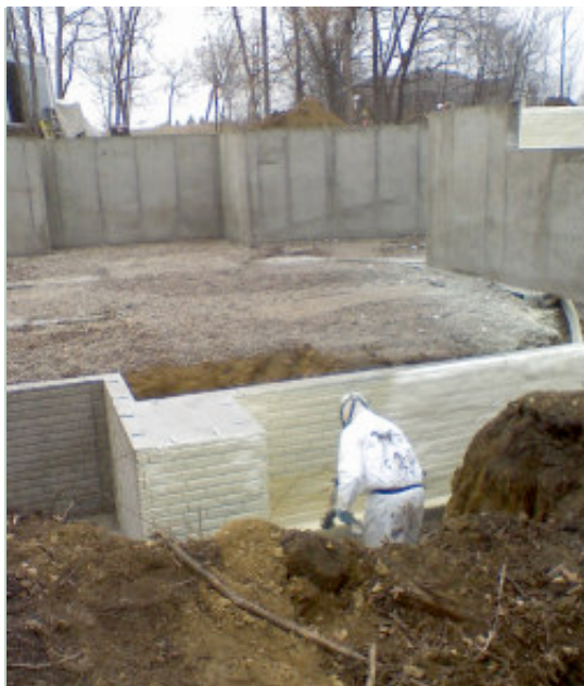
Spray polyurethane foam can be used on foundation walls and under slabs as an alternative to polystyrene.
