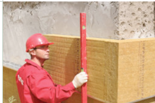
Rigid mineral wool can be an excellent substitute for polystyrene, owing to its moisture repellency and insect resistance.
