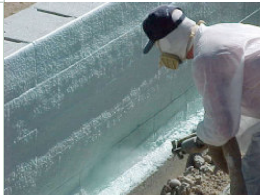
Spray polyurethane foam is becoming increasingly common as an exterior foundation insulation in Canada and northern states in the U.S. No more than 2” should be applied at a time, though multiple layers can be used to achieve very high R-values.
